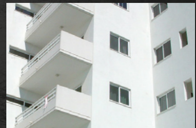
Waterproofing of exterior walls
