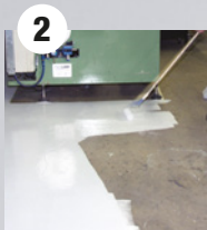
Apply 7100 floor coating
