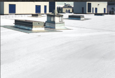
Full roof renovation
