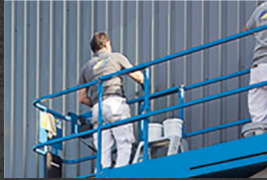
Metal cladding rejuvenation & renovation
